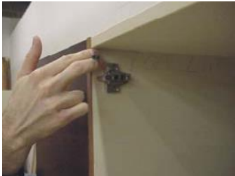
Corner Filler Panel Installation Detail
